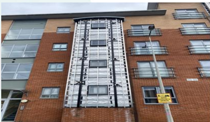
B2 Now Ready For Fire Stop & Insulation
